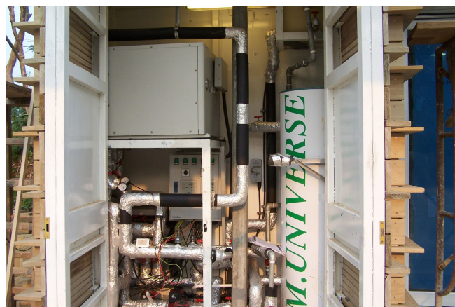
Fig. 1: An on-site photo of the project
